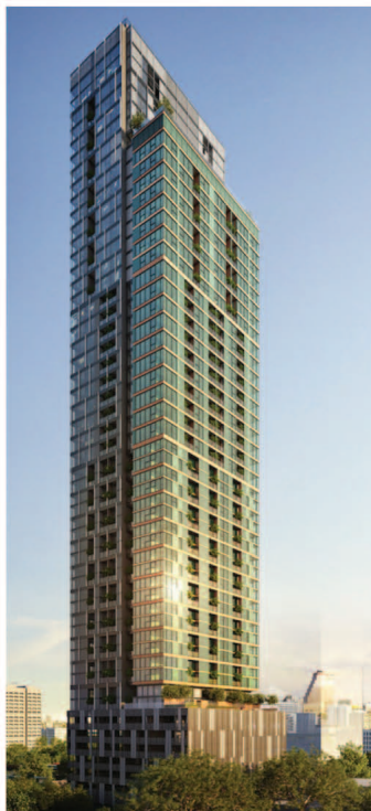
THE LOFTS SILOM-MAIN TOWER
